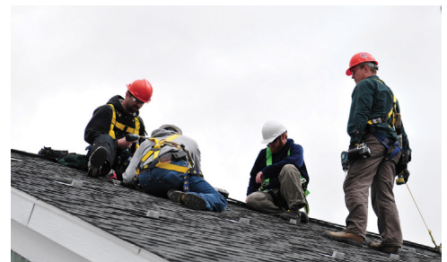
Array Standoffs Attached to the Roof’s Substructure
